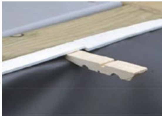
Figure 31 – Blocking the liner in position using half clothes pegs
