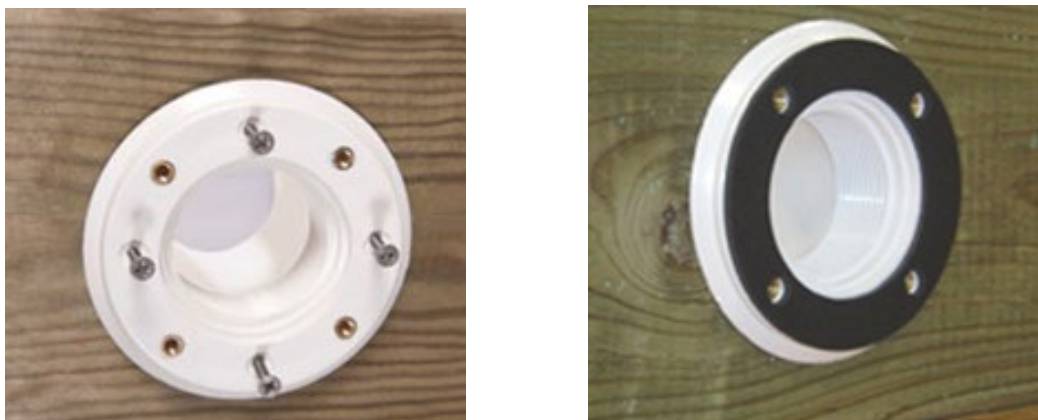
Figure 23 – Mounting the return fitting body and gasket
