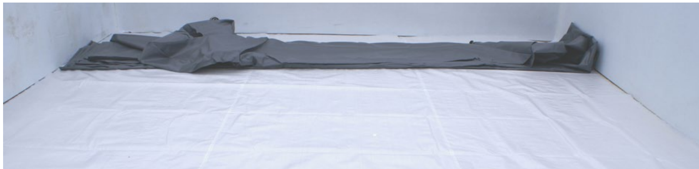
Figure 32 – Unfolding the liner
