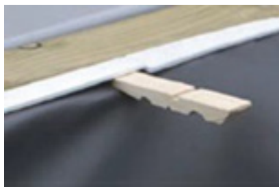
Figure 28 – Blocking the liner in position using half clothes pegs
