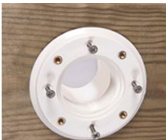
Figure 24 – Mounting the return fitting body and gasket
