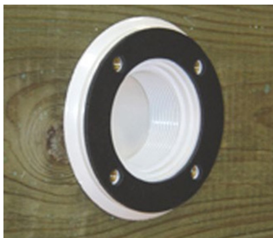
Figure 24 – Mounting the return fitting body and gasket
