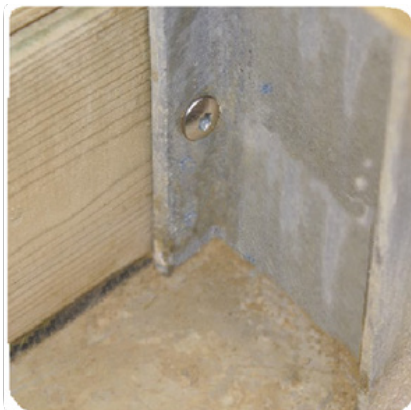
Figure 9 – Fastening the slats to the supporting braces
