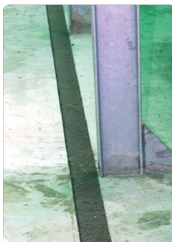
Figure 7 – Laying the bituminous strips
